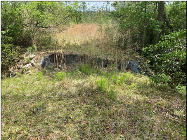
PHOTO 9. VIEW LOOKING SOUTH SHOWING 2 – 48-INCH CULVERTS (DAMAGED) AT STREAM FSI NEAR ROAD #3A (MAY 2021).
