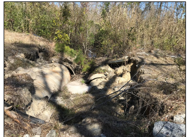
PHOTO 12. VIEW LOOKING NORTHWEST ALONG STREAM FSI SHOWING 2 – 48-INCH CULVERTS (DAMAGED) AT ROAD #6 CROSSING NEAR PROPERTY LINE .
